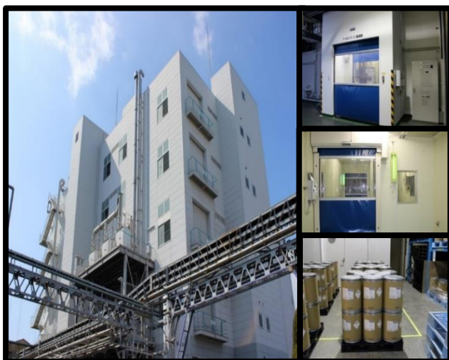
Izumi Factory's manufacturing building (Izumiotu City, Osaka)
