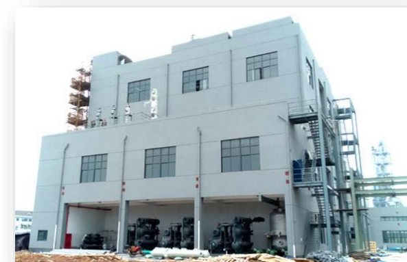
Quzhou BDX New Chemical Materials Co., Ltd. (China)
