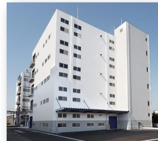
Izumi Factory's manufacturing building (Izumiotu City, Osaka)
