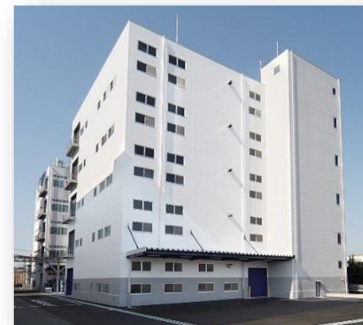
Izumi Factory's manufacturing building (Izumiotu City, Osaka)
