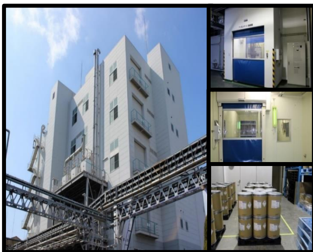
Izumi Factory's manufacturing building (Izumiotu City, Osaka)
