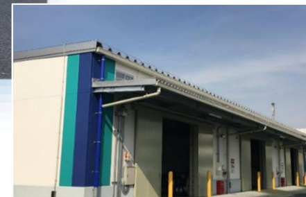
Headquarters new hazardous materials warehouse (completed in December 2018)
