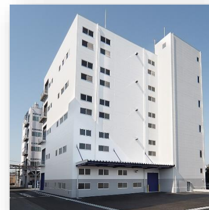
Izumi Factory's manufacturing building (Izumiotu City, Osaka)
