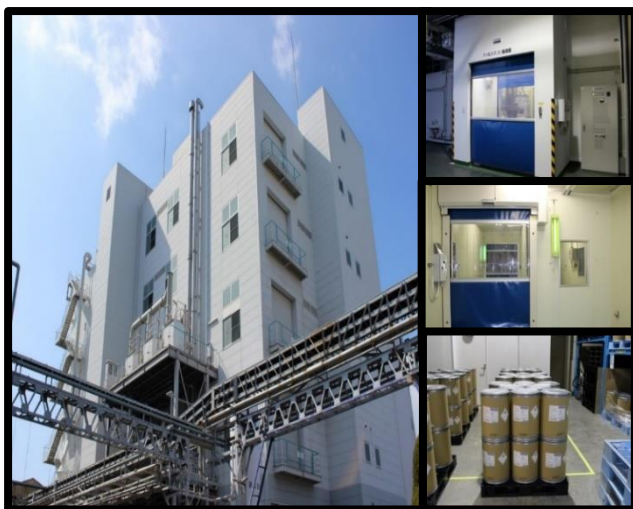
Izumi Factory's manufacturing building (Izumiotu City, Osaka)
