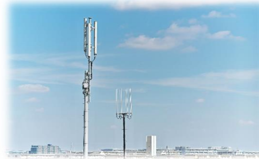
Deployment to communication infrastructure
