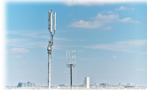
Deployment to communication infrastructure
