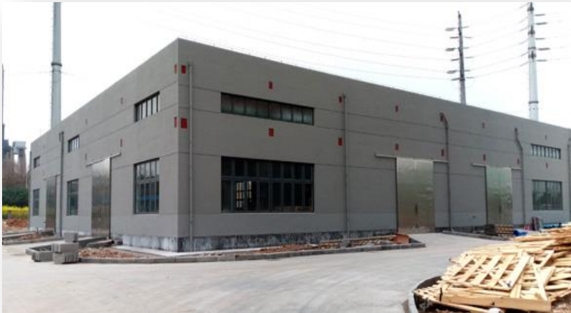
Product and material warehouse
