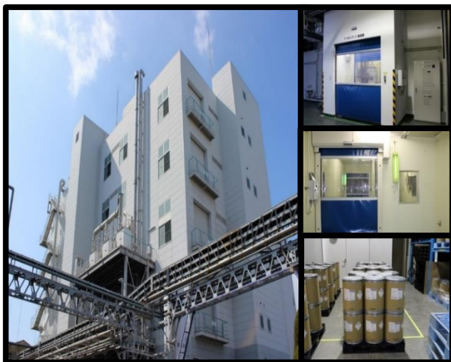
Izumi Factory's manufacturing building (Izumiotu City, Osaka)
