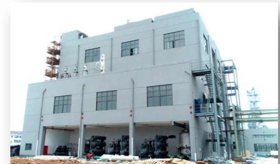
Quzhou BDX New Chemical Materials Co., Ltd. (China)
