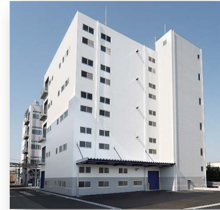
Izumi Factory's manufacturing building (Izumiotsu City, Osaka)
