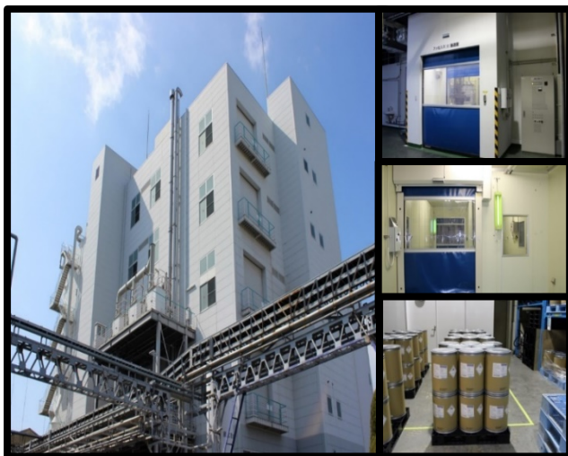
Izumi Factory's manufacturing building (Izumiotu City, Osaka)
