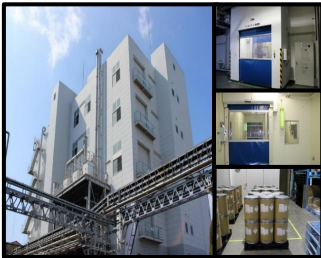
Izumi Factory's manufacturing building (Izumitsu City, Osaka)
