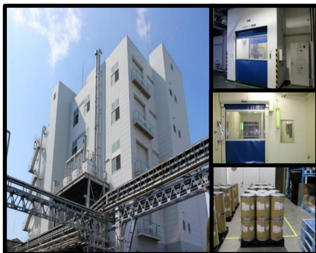
Izumi Factory's manufacturing building (Izumiotu City, Osaka)
