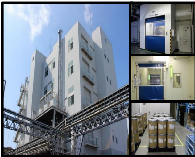
Izumi Factory's manufacturing building (Izumitsu City, Osaka)
