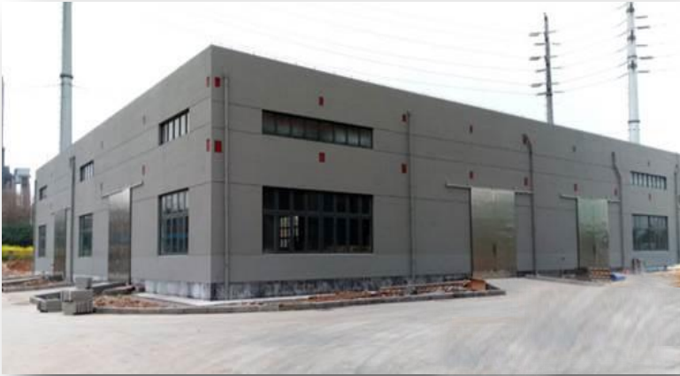
Product and material warehouse
